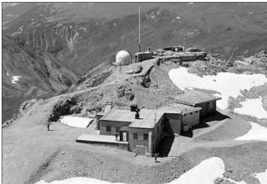
Radar meteorologic sin in Weissfluh.
